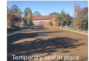
Temporary seal in place
