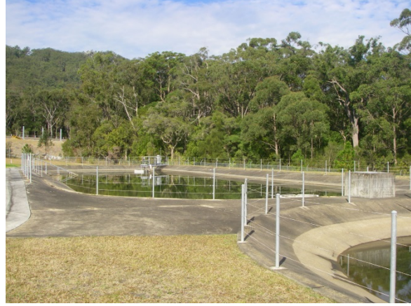
Figure 24: Bulahdelah WTP sludge lagoons
