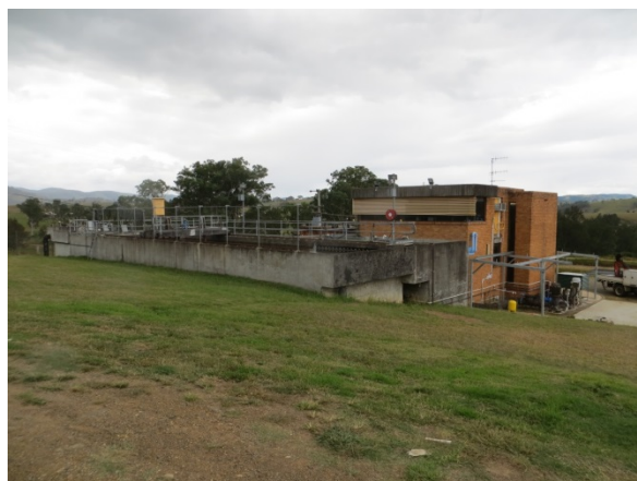
Figure 42: Gloucester WTP buildings
