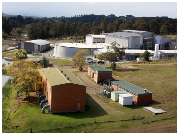
Figure 14: Old treatment building in foreground
