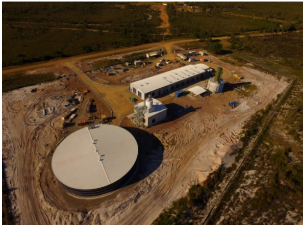
Figure 6: Nabic WTP during construction
