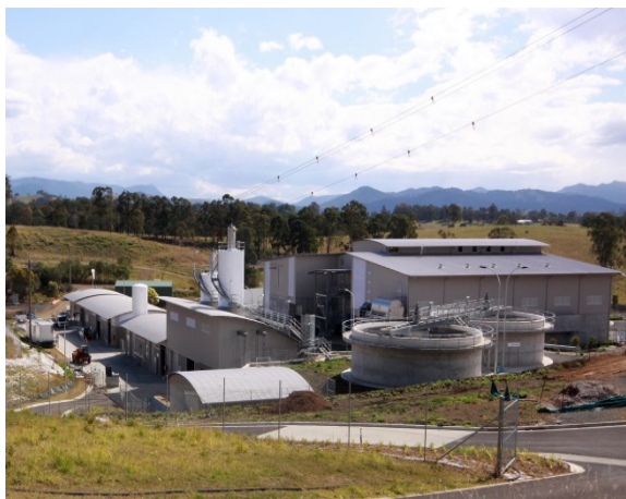
Figure 13: Bootawa WTP and laboratory
