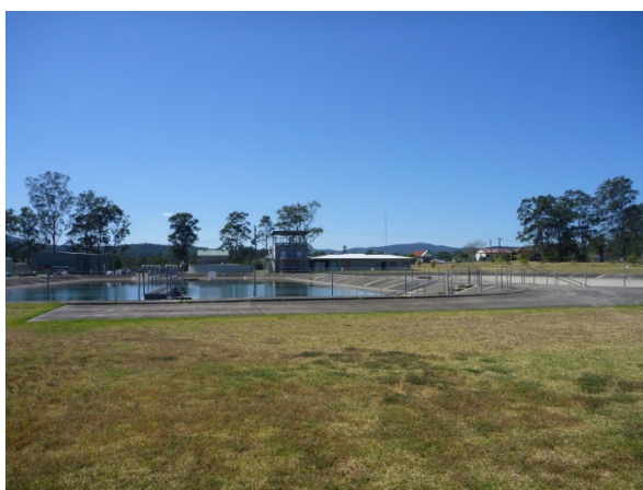
Figure 30: Stroud settling lagoons
