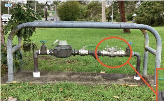
A 50mm water meter with a backflow prevention device to prevent potential contamination
