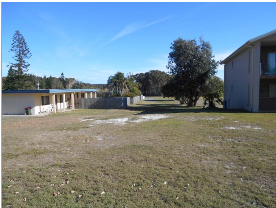
Figure 6.5 Existing holiday units and house facing west
