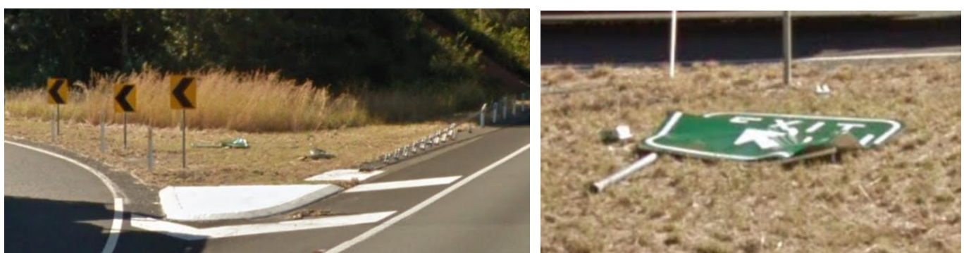
Figure 8-2: Google Map Images of Damaged Sign and Wire Rope Fence on Nthb Exit Ramp
