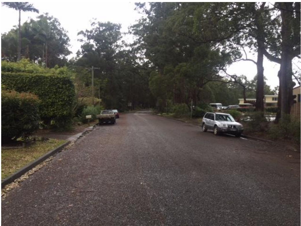
Photo No. 6: Looking generally south along Kolodong Road showing the existing traffic environment past the Taree Christian College towards the end of the existing sealed pavement.
