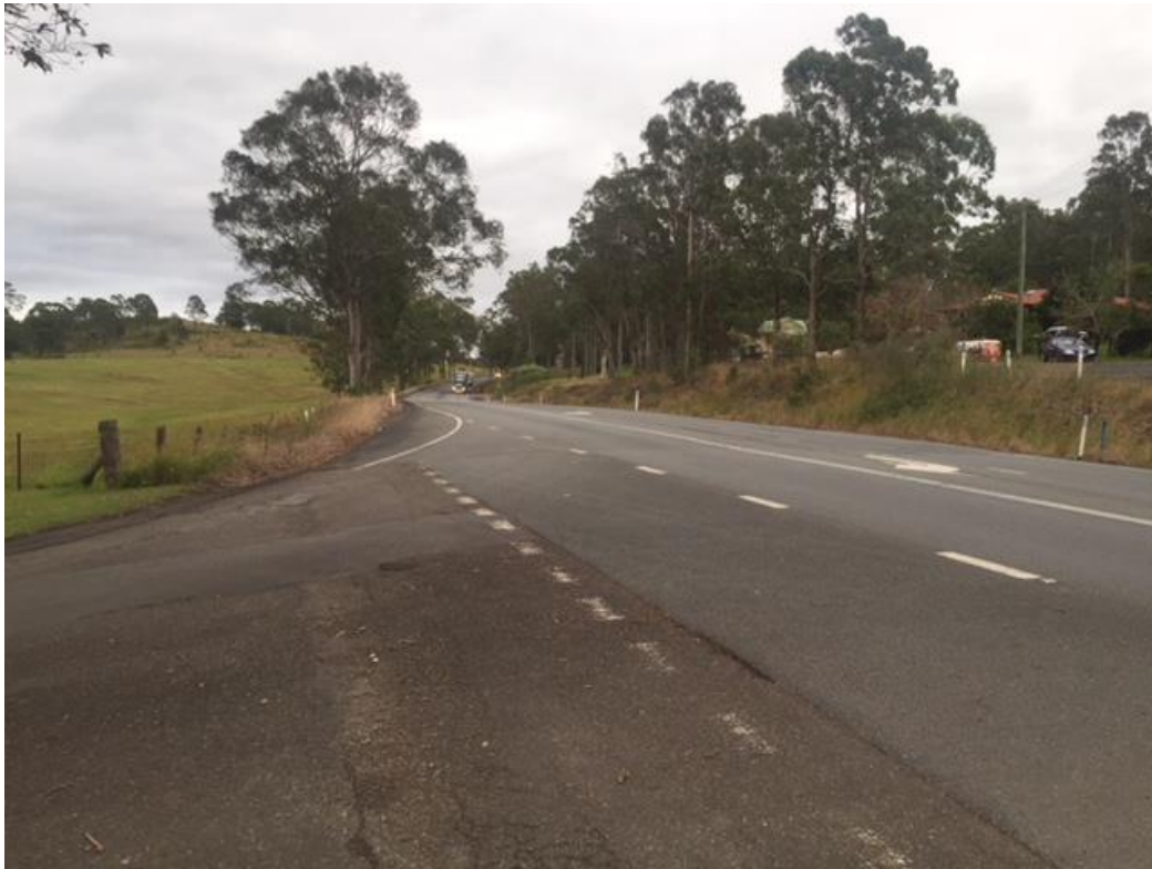
Photo No. 1: Looking left (generally west) along Wingham Road from Kolodong Road showing the existing traffic environment and sight distances.
