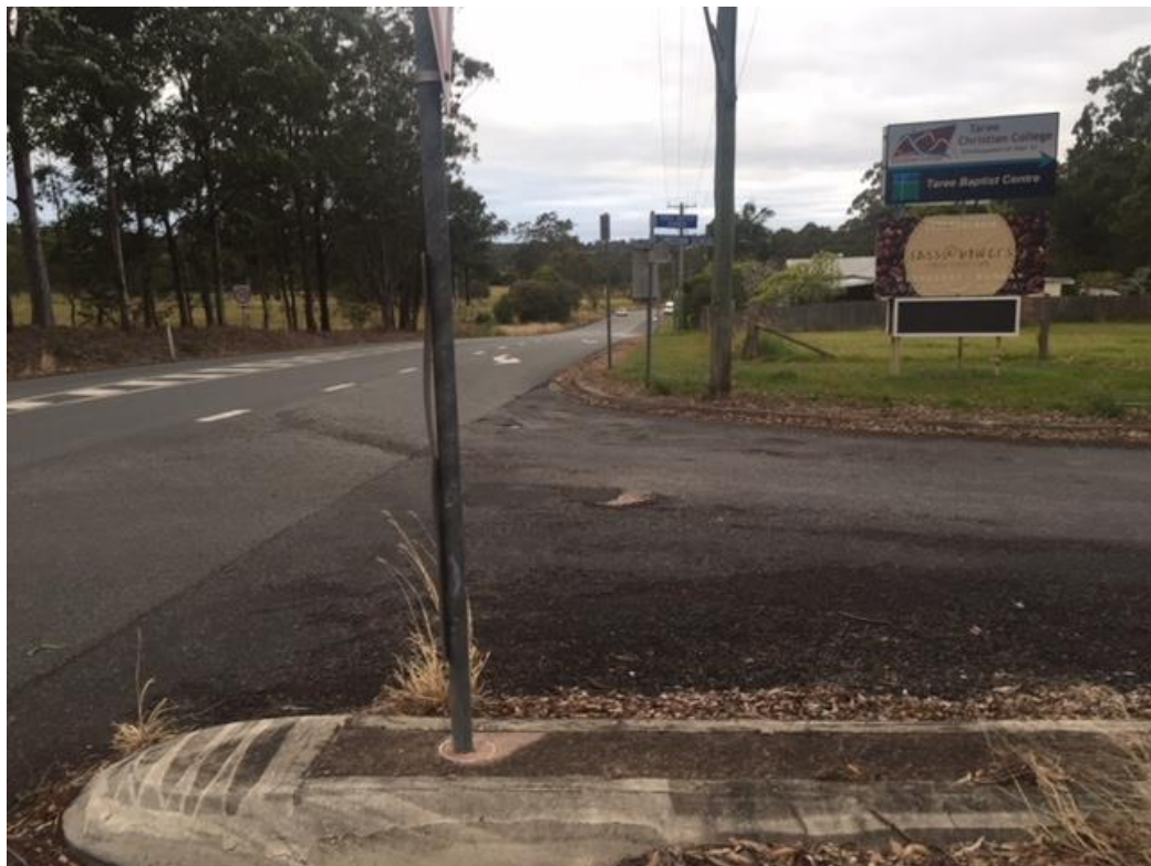
Photo No. 2: Looking right (generally east) along Wingham Road from Kolodong Road showing the existing traffic environment and sight distances.
