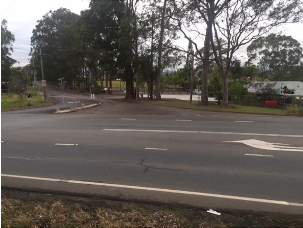
Photo No. 3: Looking generally south along Kolodong Road from Wingham Road showing the existing traffic environment.
