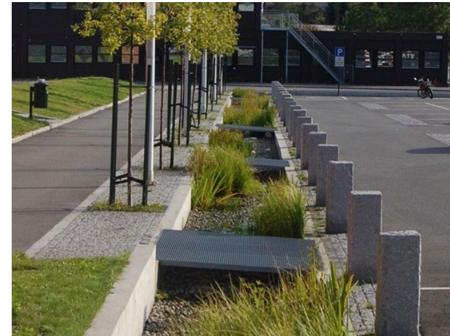
13 Chapman parking upgrades with water sensitive urban design
