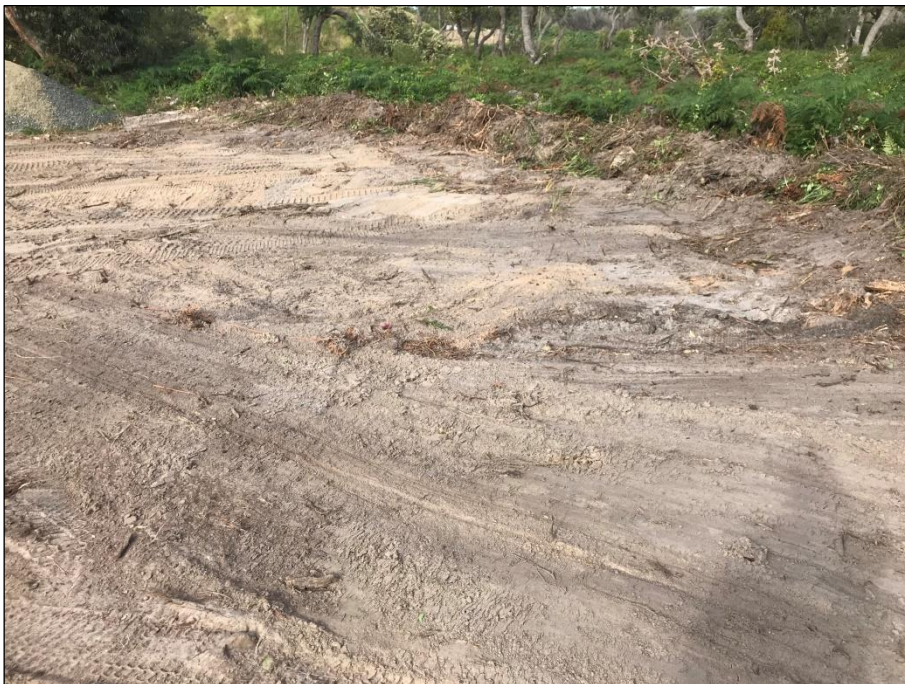
Figure 6: Clearing/grading of the surface in the western portion of the site, looking south
