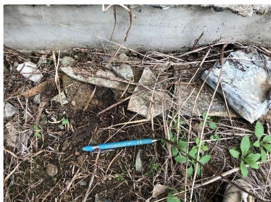
Fragments of fibro-cement sheeting suspected as being ACM on the ground surface up against the northern side of the shed on lot 50. ACM sample ACM1 was collected from this location.
