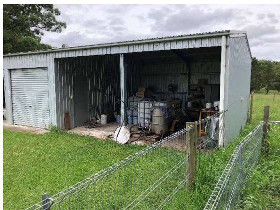
Looking southwest showing a shed with stored drums and containers of unknown liquids located on the southern side of the house in the central part of Lot 2 DP827097.
