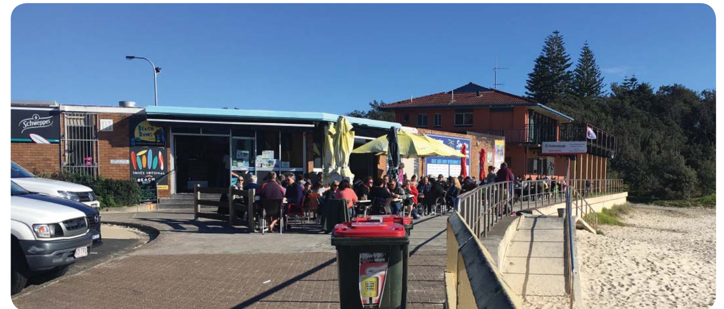
(top): The southern facade of the existing building (bottom): The beach side facade of the existing building
