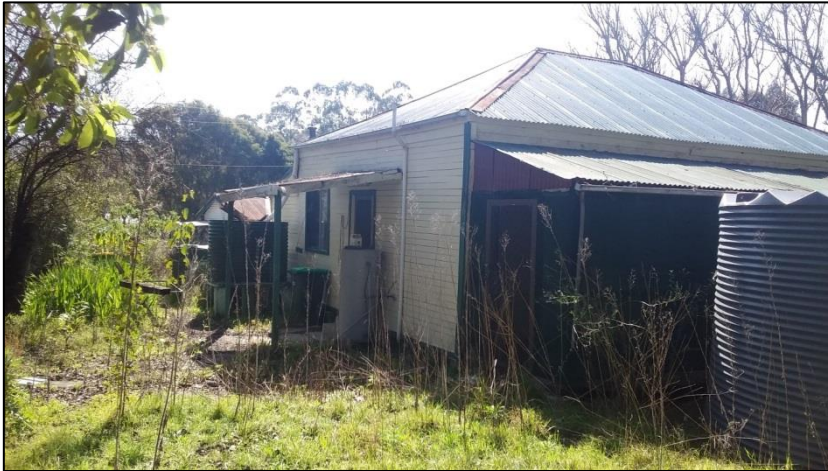
Figure 4: Existing residence in Lot 9, looking north-west
