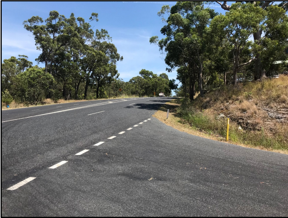
Photo 1 - Myall Way looking right (west) from Viney Creek Road East showing sight distance
