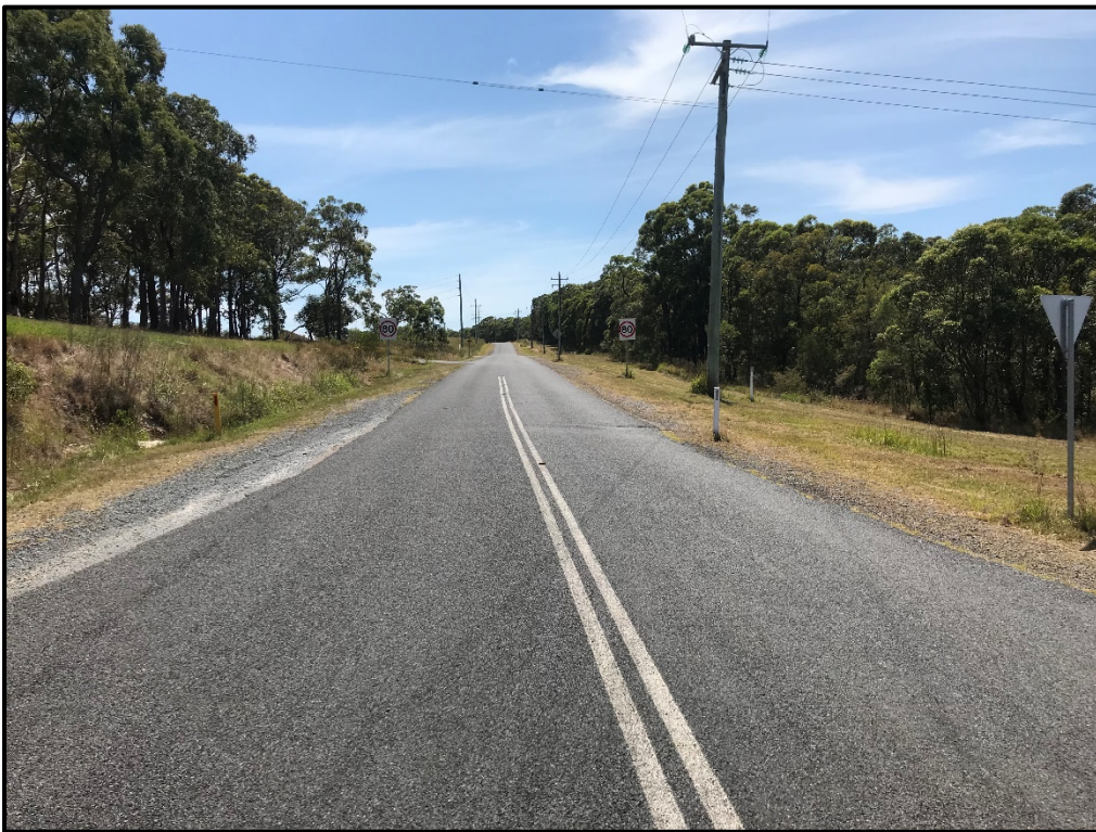
Photo 4 - Cross section of Viney Creek Road East to the north of the intersection with Myall Way/Tea Gardens Road
