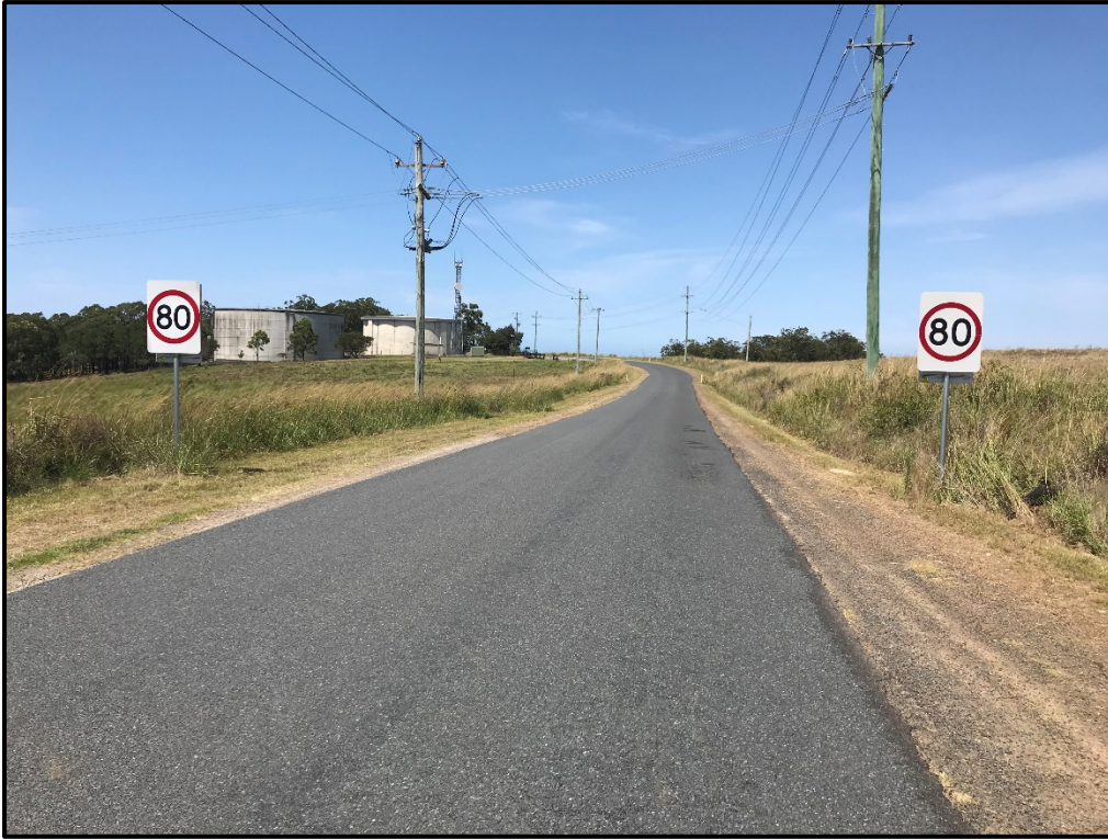
Photo 3 - Cross section of Viney Creek Road East looking southbound (Subject site located on the right)
