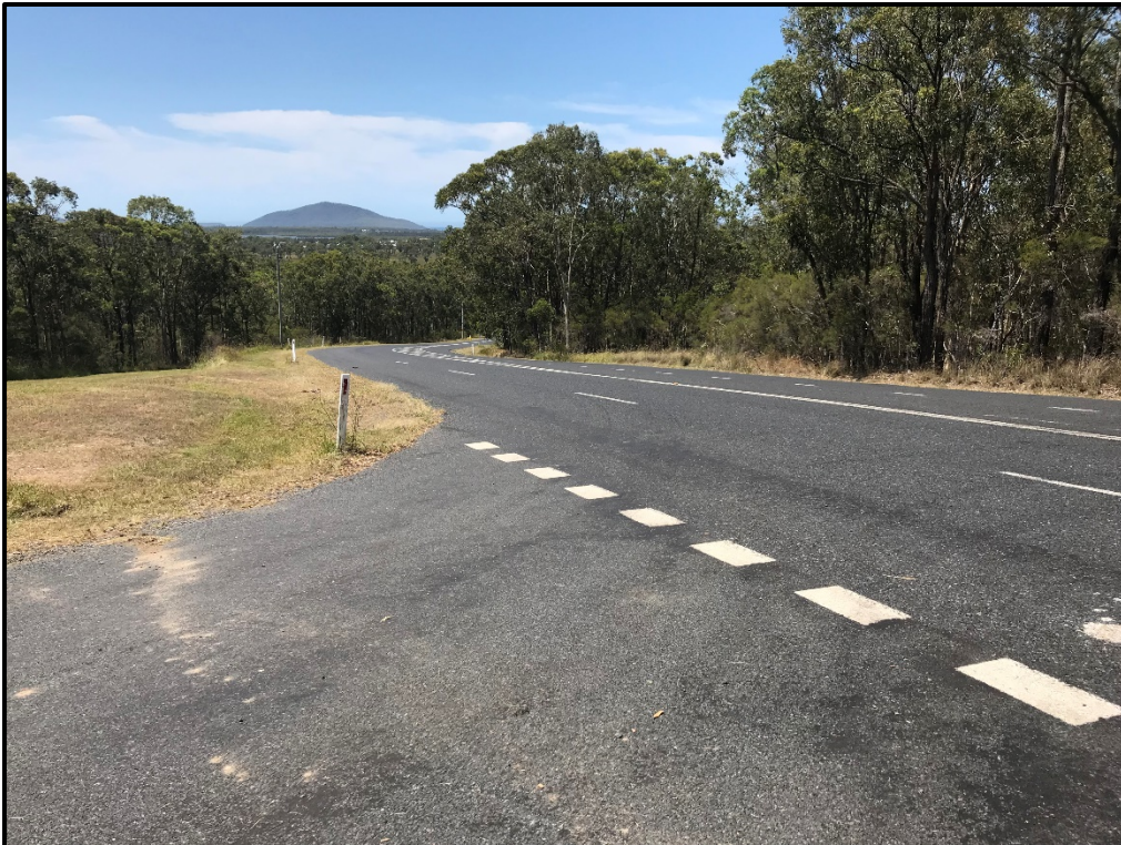
Photo 2 Myall Way looking left (east) from Viney Creek Road East showing sight distance
