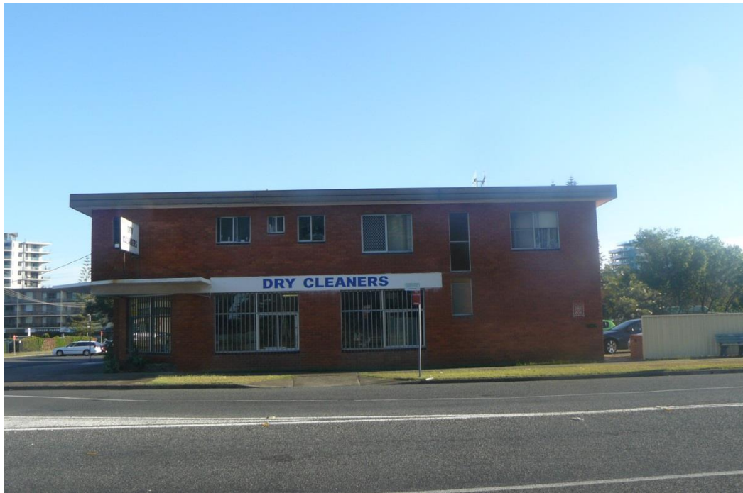
Existing commercial building opposite site
