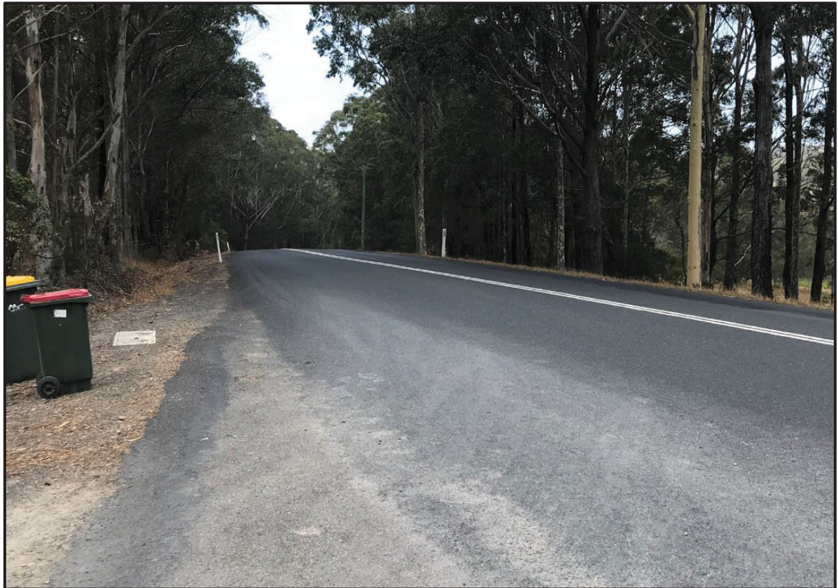
Photo 4 - View to left for a driver exiting the access road onto Coomba Road
