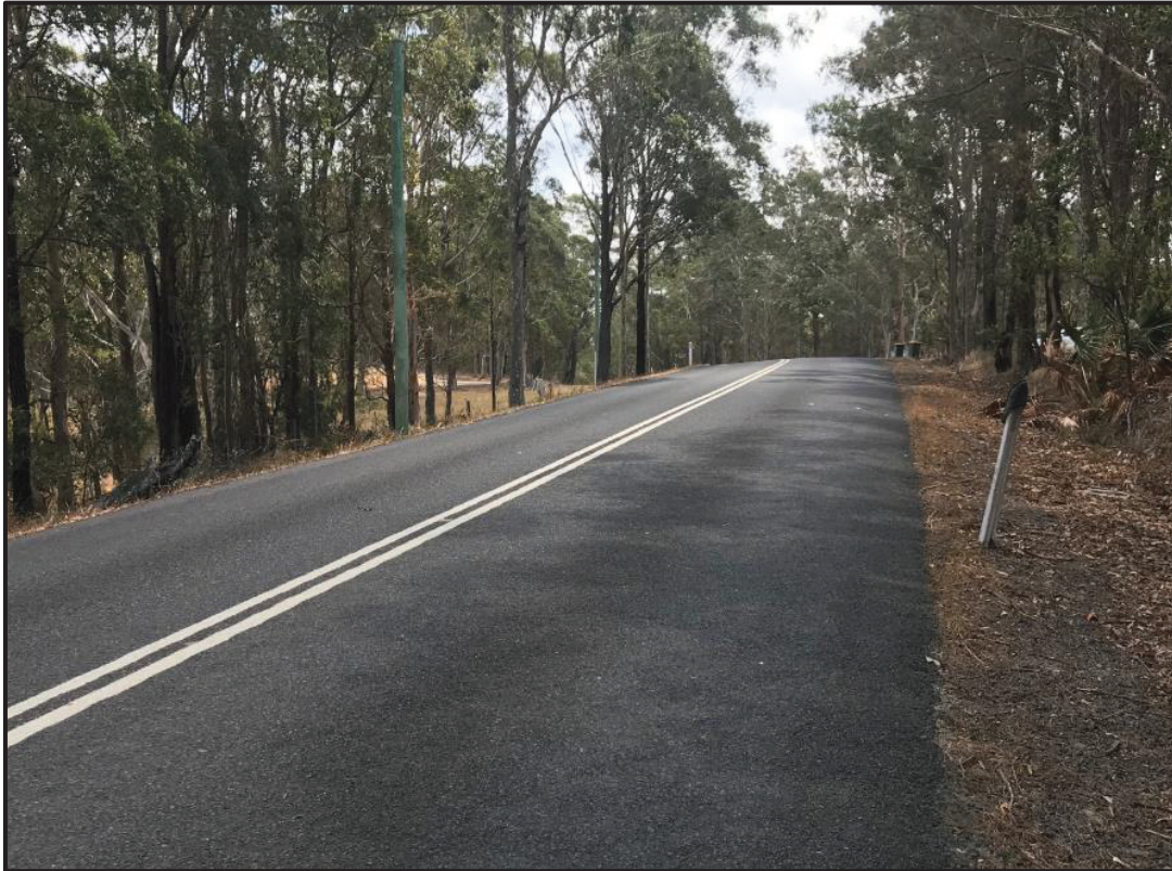
Photo 1 – View along Coomba Road showing typical cross section in vicinity of the subject site.
