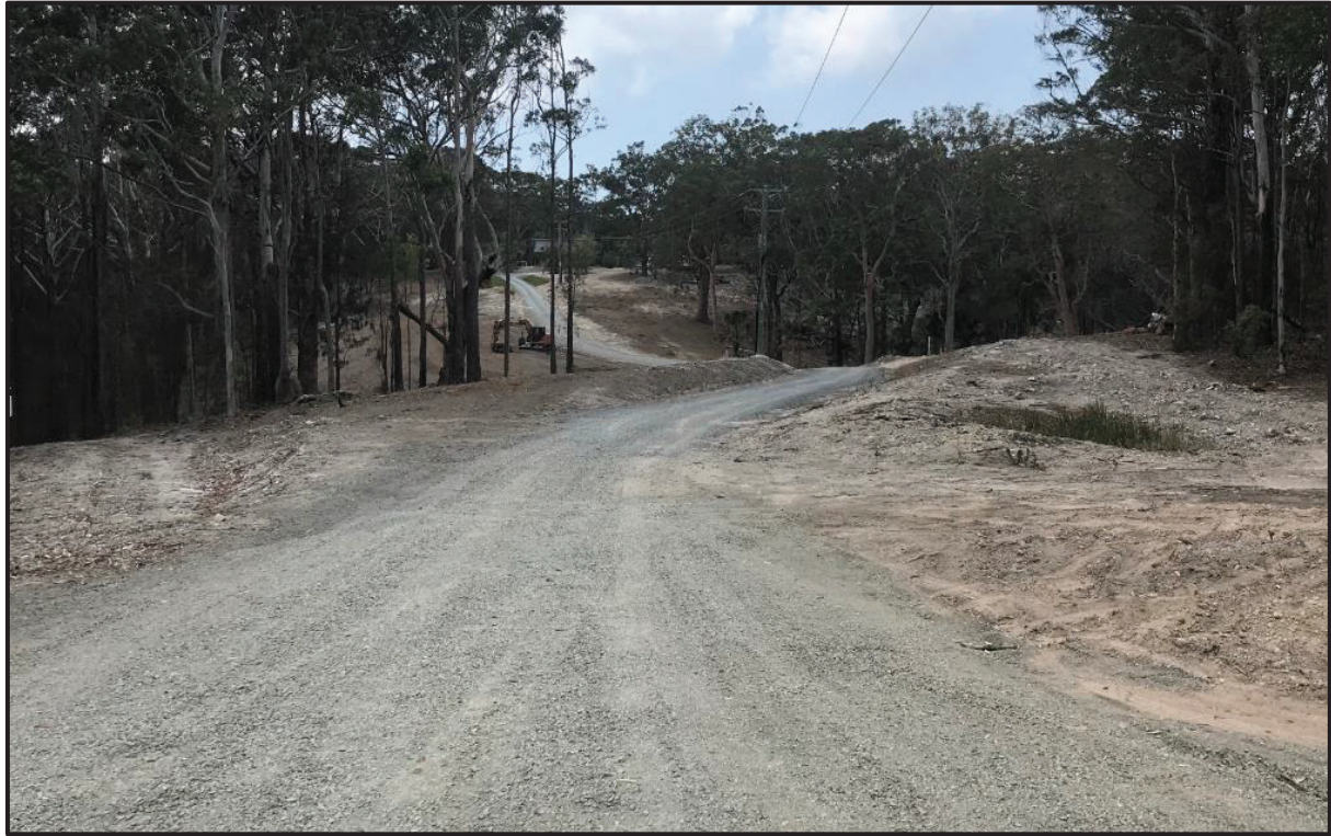
Photo 2 – View along access driveway to 96 Coomba Road showing typical cross section and alignment
