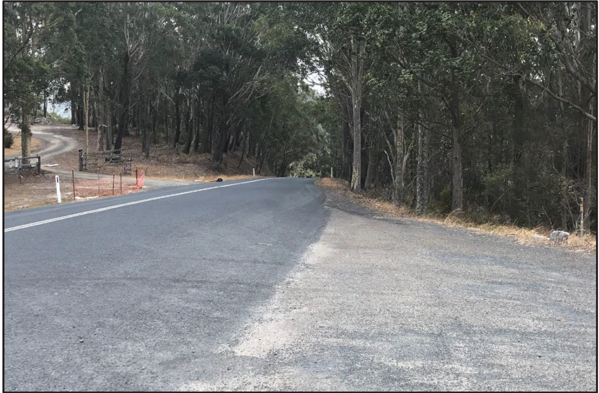
Photo 3 – vView to right for a driver exiting the access road onto Coomba Road
