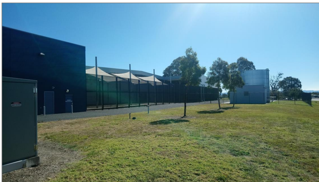
Photograph 1 - East Elevation (Frontage to Manning River Drive)
