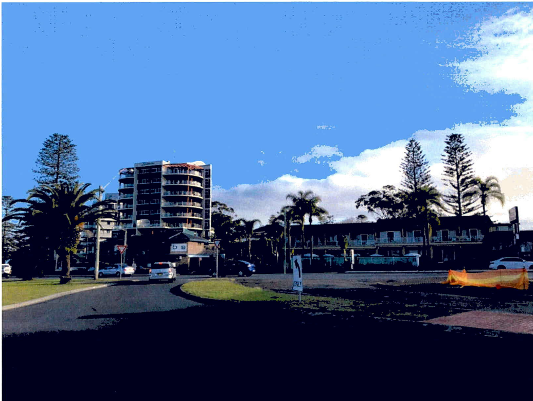
Residential tower on Manning Street and motel approved for 10 storey mixed use building
