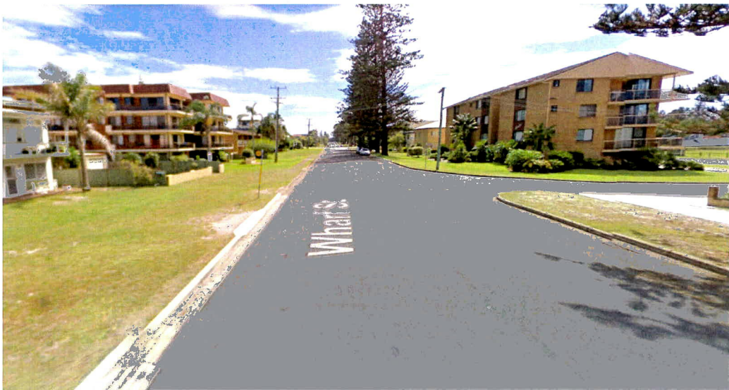
Existing residential flat buildings along Wharf Street, Tuncurry
