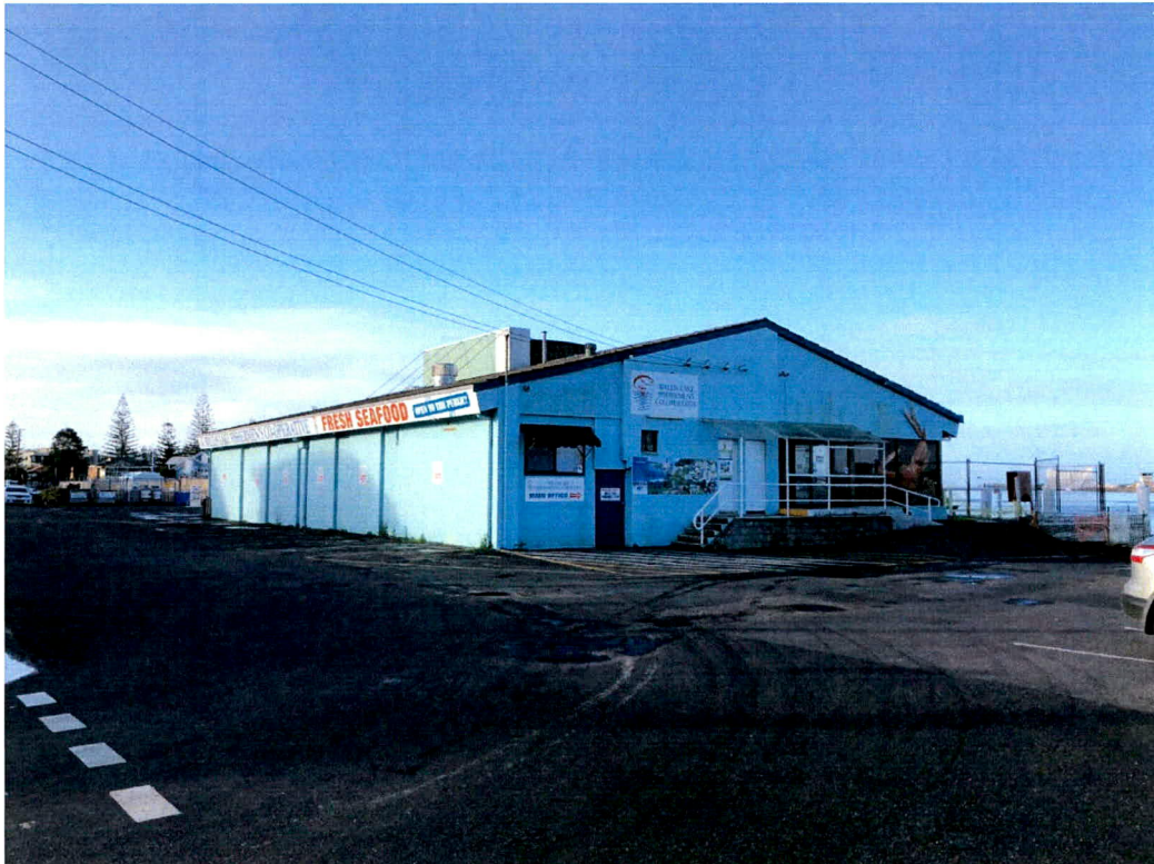
Existing Fish Cooperative building opposite on Leo Amato Close
