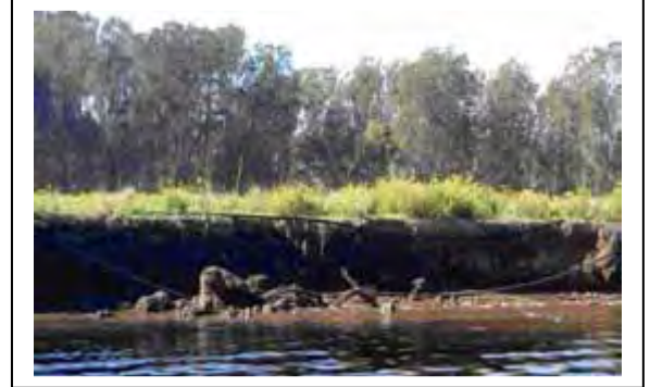
Bank Erosion on the lower Wallamba River
