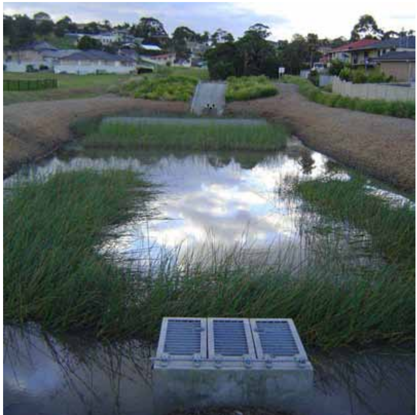
Figure 17. Pioneer constructed wetland - designed to remove pollutants before draining into Wallis Lake
