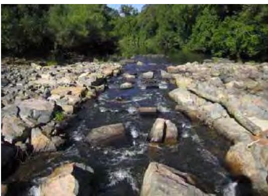
Figure 20. Modifications to the Stroud Water Supply Weir to allow fish movement. Source: DPI (Fisheries)
