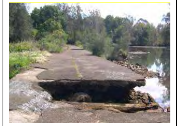
The derelict causeway on the Wallamba River at Clarksons Crossing
