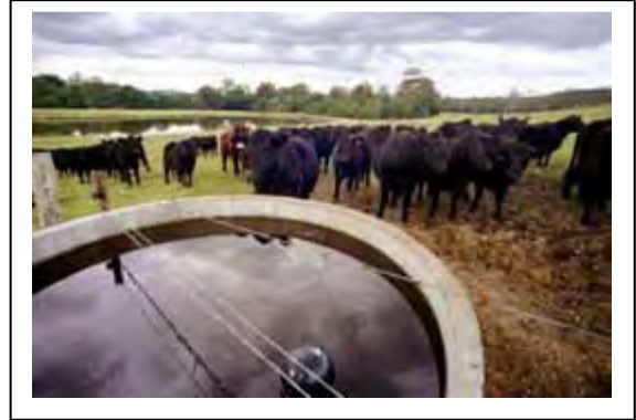
Off-stream stock watering system installed to rehabilitate and protect the riparian zone
