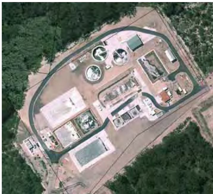
Figure 44. Sewage treatment at MidCoast Water's Hallidays Point sewage treatment plant.
