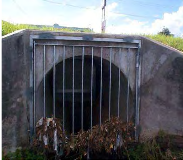
Figure 18. Gross Pollutant Traps, like the one in Little St, remove large debris
