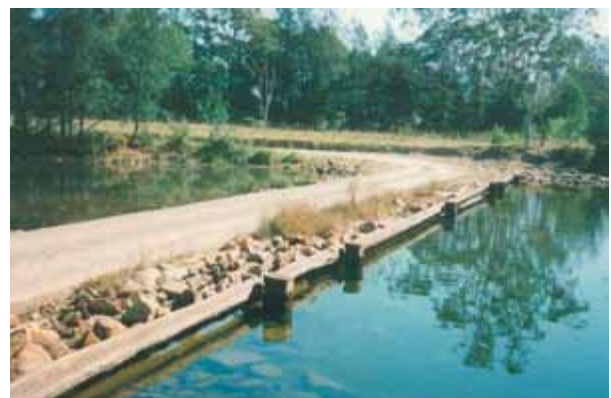
Locketts Crossing – a physical barrier that restricts fish migrations.
