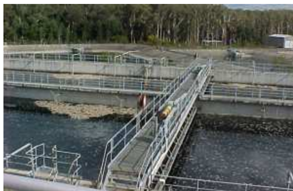
Sewage treatment at MidCoast Waters Forster sewage treatment plant.
