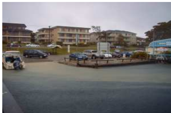
Erosion caused by a rain event whereby sediment is washed into local waterways, in this case Wallis Lake
