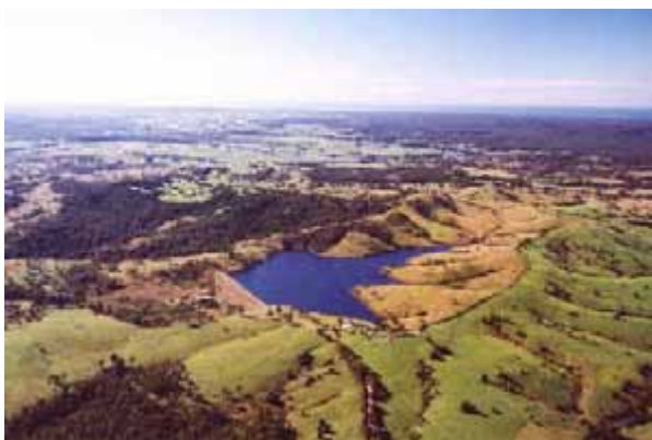
Bootawa Dam: the main storage area for the Manning water supply scheme.
