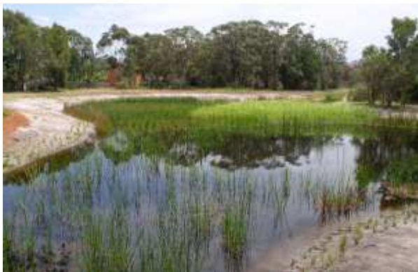
Goldens Road South constructed wetland – designed to remove pollutants before draining into Wallis Lake.
