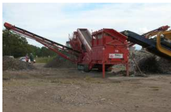
Concrete crushing (recycling into roadbase) – Tuncurry waste management centre
