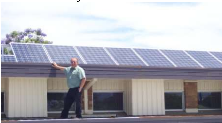
Photo 15: Solar panels on the roof of the Council buildings.
