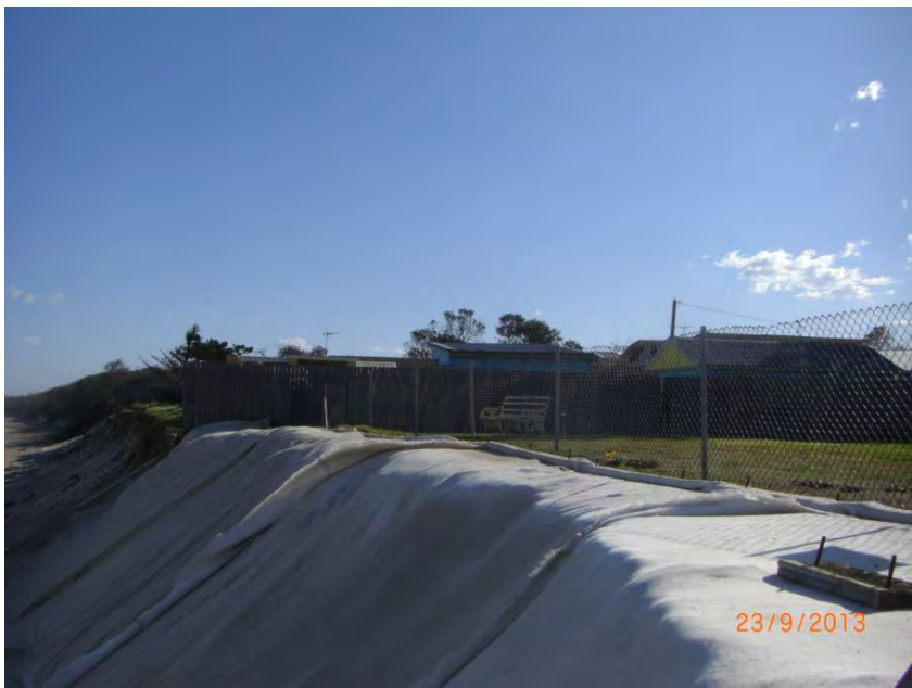
Photo 23 – Geotextile “wall” opposite Meridian Resort
