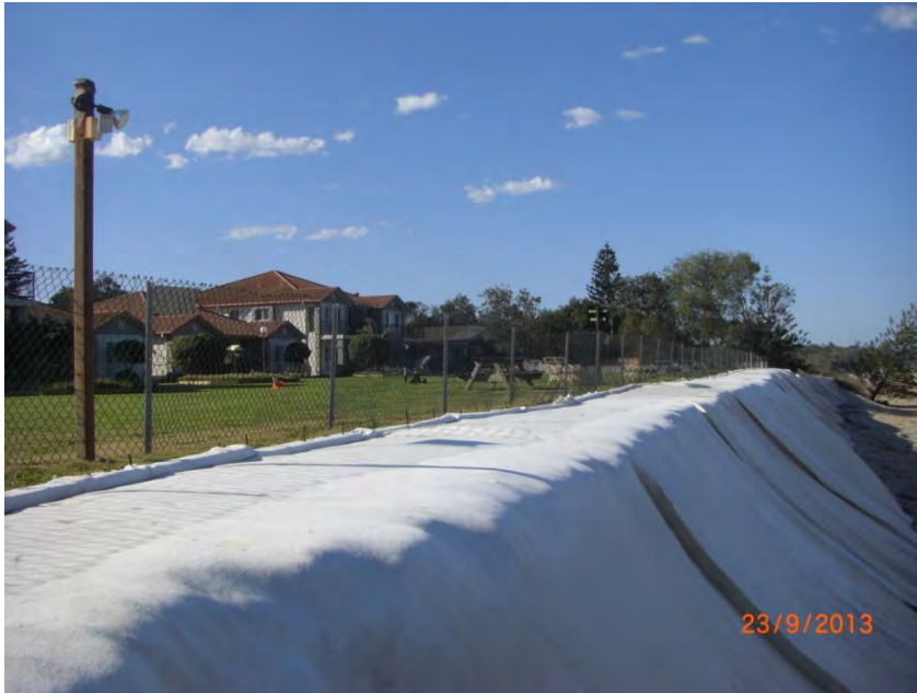
Photo 24 - Geotextile "wall" opposite Meridian Resort
