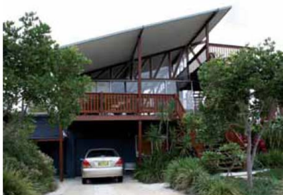
Raised, lightweight structure allows for undercroft parking; clerestory allows sunlight from the east and view to the coast
