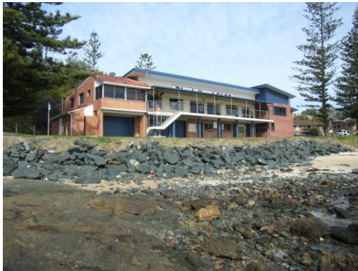
Rock protection around Black Head SLSC
