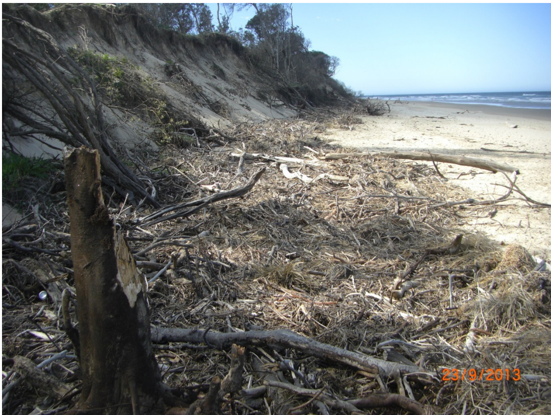
Photo 1 – Loss of dunes and vegetation between the school and entrance to Racecourse Creek
