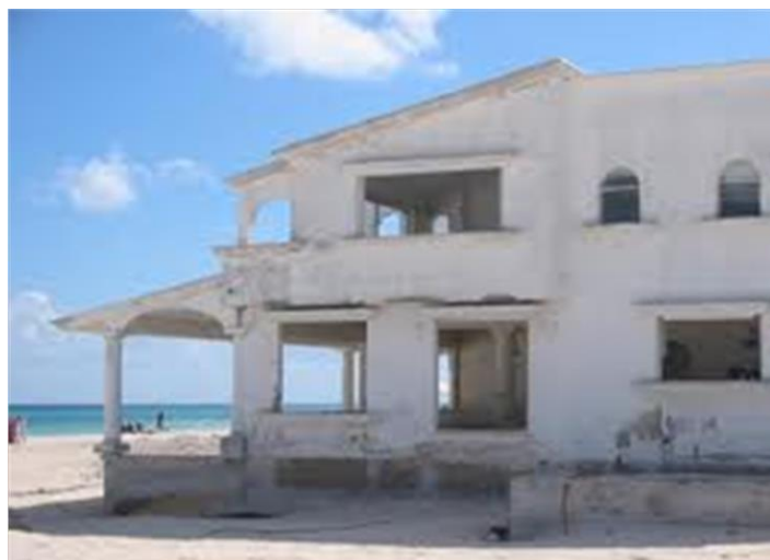
House intended for demolition after abandonment, USA
