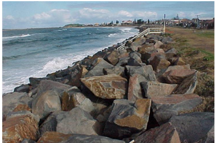
Rock seawall at Stockton Beach, Newcastle, showing the lack of beach at high tide.
