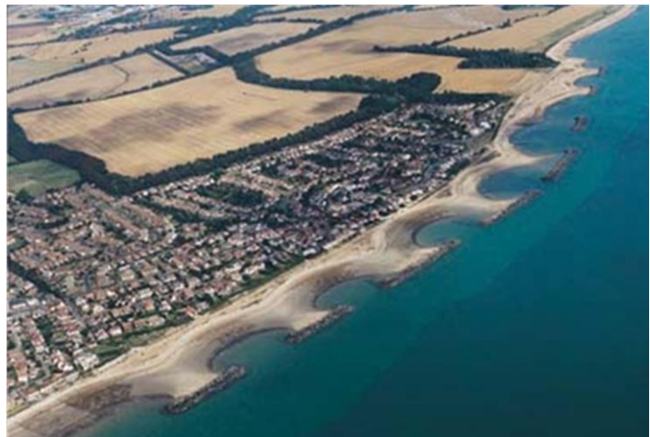
Example emergent breakwater in UK, where the lower energy environment is more suited to such options
