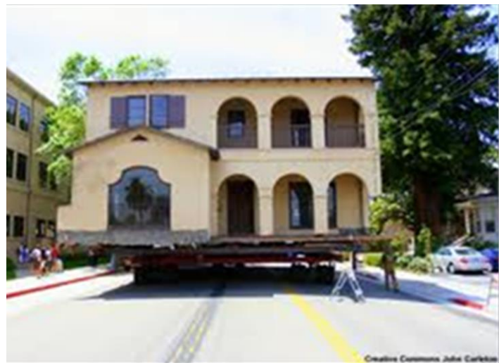
House being relocated out of hazard area
