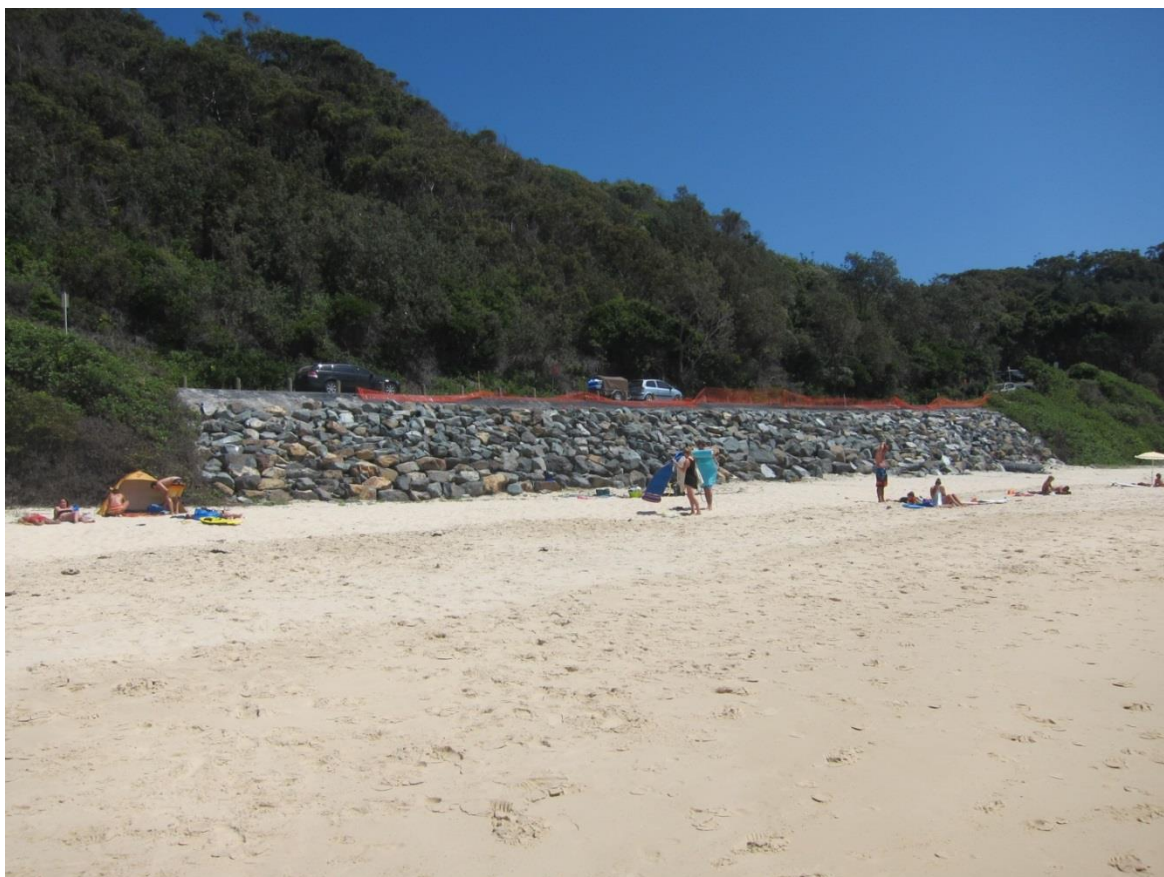
Figure 2-2 Rock revetment recently constructed to manage landslide risks to Seal Rocks Road, Number One Beach
