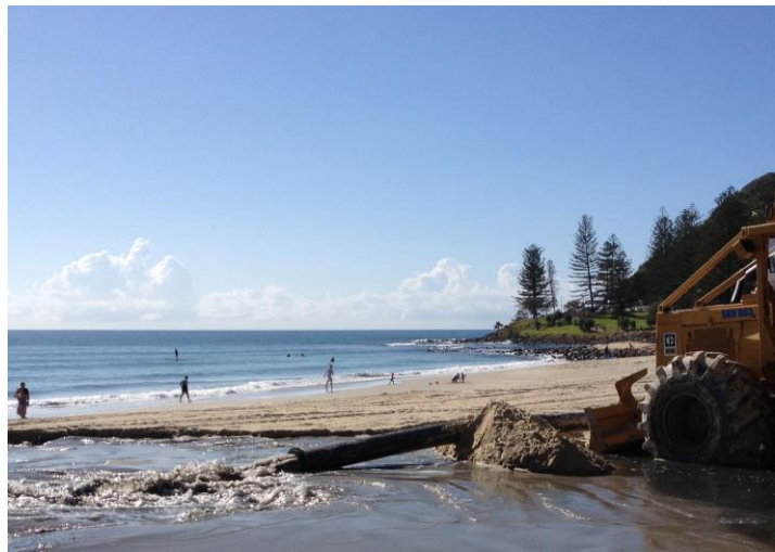
Nourishment of beach with sand at Burleigh Heads, Qld.
