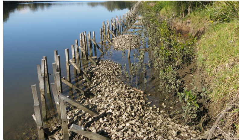
Figure 30: Erosion on the riverbank following installation of the Oyster Reef
