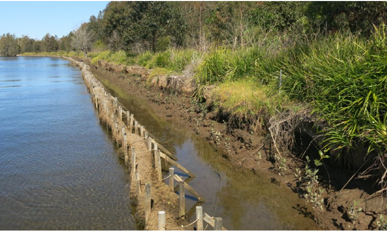
Figure 29: Erosion on the riverbank prior to installation of the Oyster Reef
