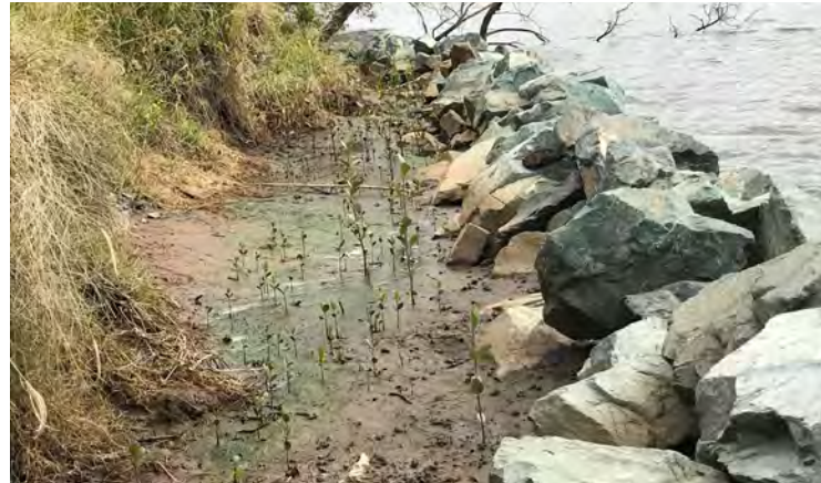
Figure 30: Mangroves regenerating behind rock fillets to protect the bank from erosion on Dumaresq Island
