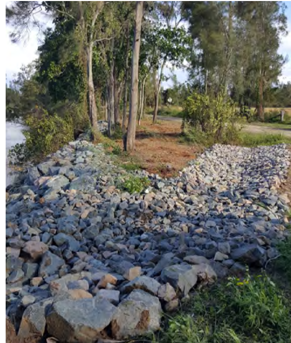
Figure 33: Completed erosion and sediment controls on North Moto Road undertaken as part of the Marine Estate Management Strategy Program
