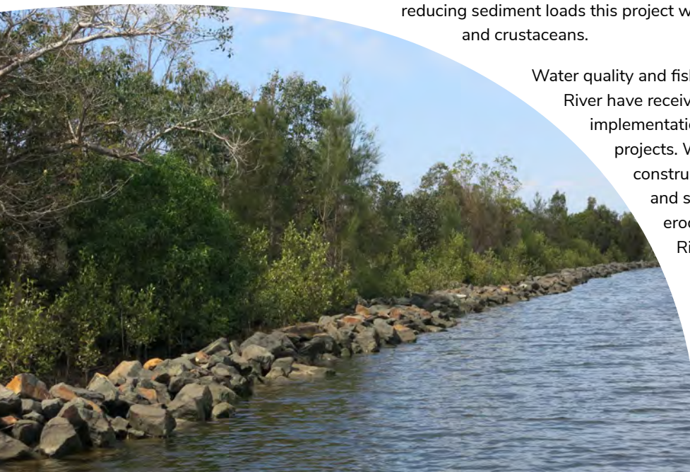
Figure 38: Bank stabilisation works in the Wallamba River
