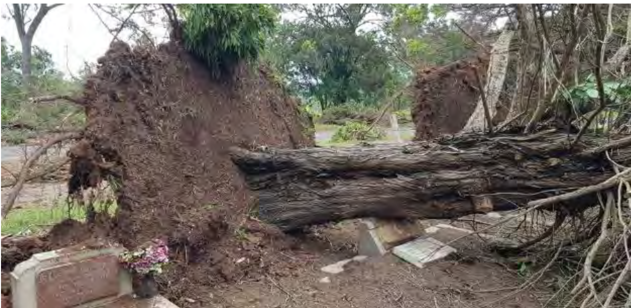
Plate 4.16 Detailed view of damage to grave markers as a result of fallen trees, December 2018
