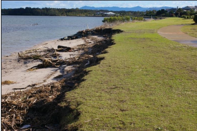
Above: Eroding riverbank at Harrington Waters
