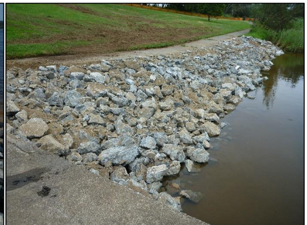
Above: Manning Waters Rock Revetment
