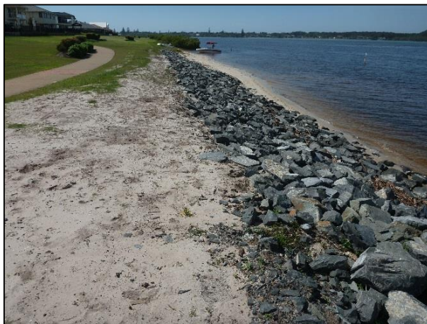
Above: Harrington Waters Rock Revetment
