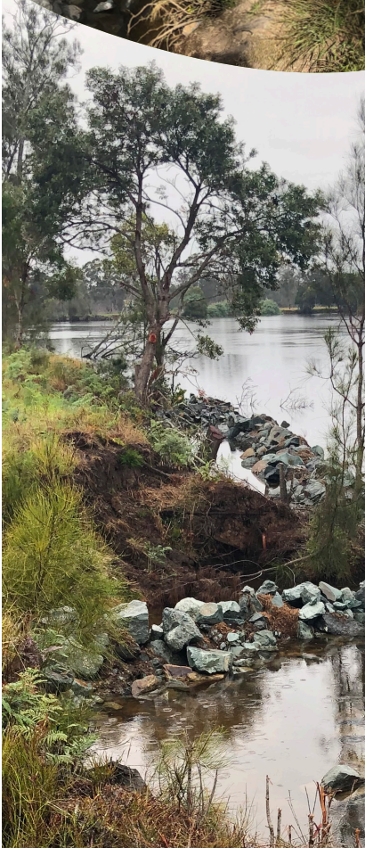
Extensive rock fillet works at stock exclusion fencing have been installed along the Wallamba River.
