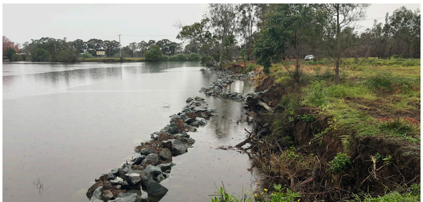
Extensive rock fillet works at stock exclusion fencing have been installed along the Wallamba River.
