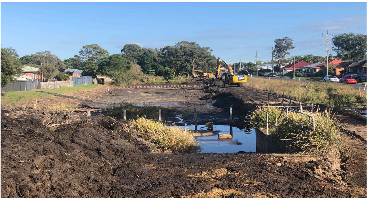
Townsend Wetland during construction
