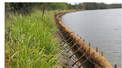
Biodegradable Coir Logs provide erosion control and help mangroves establish stabilising the bank.
