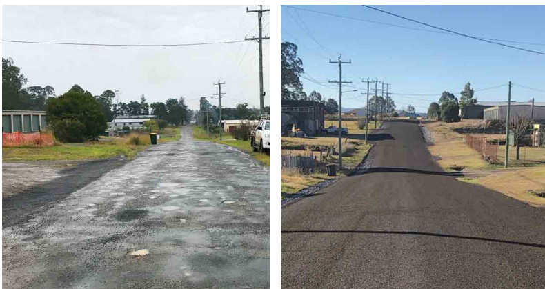
Britten Street, before (left) and after (right)
