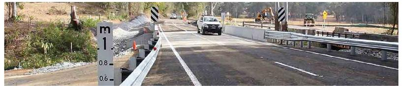
The recently reconstructed Milbai Creek Bridge, Tinonee is a two lane concrete bridge designed to modern loadings. It provides a wider, safer and more seamless thoroughfare for local traffic.
