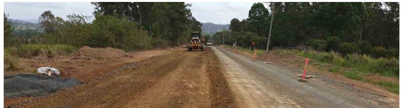
A 630m stretch of busy Avalon Road at Krumbach connecting travellers between Gloucester and the Pacific Highway, was targeted for reconstruction. The project which is nearing completion includes widening of lanes and construction of the additional road width, a full reconstruction of the existing road pavement, line-marking, and installation of signage for improved safety.
