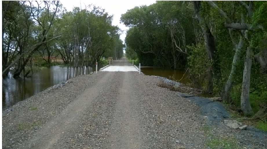
Pelican Bay Road Bridge Replacement
