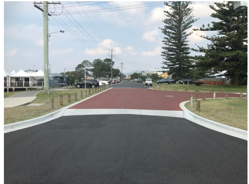
Marine Drive Roadworks
