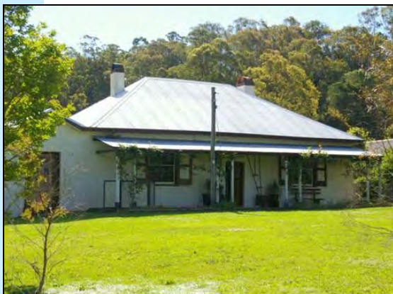
Figure 2: Early Australian Agricultural (AA) Company Cottage. The traditional roof has a simple form and the colour is not overly bright or intrusive.
