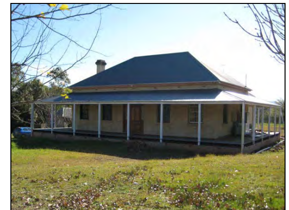
Figure 1: An excellent example of a simple, gabled corrugated iron roof. Pitch is at least 30 degrees and the colour blends in with the surrounding environment.
