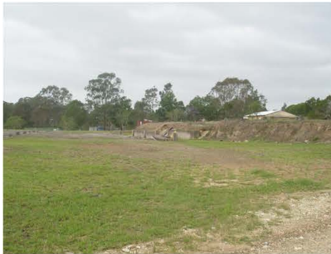
5. LOOKING SOUTH ACROSS THE REMAINING TIMBER MILL REMAINS FROM LOT 4
