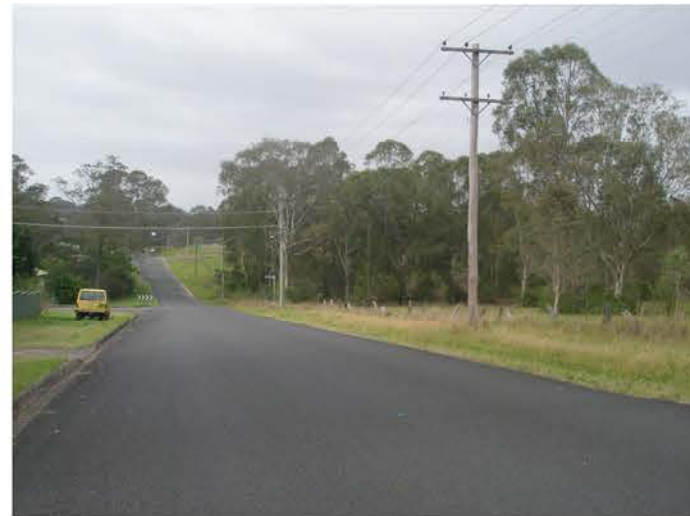
4. LOOKING SOUTH DOWN LAMBERT STREET
