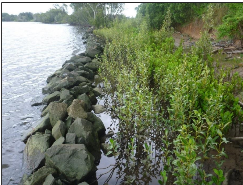
Figure 20 - River bank stabilisation along the Manning River
