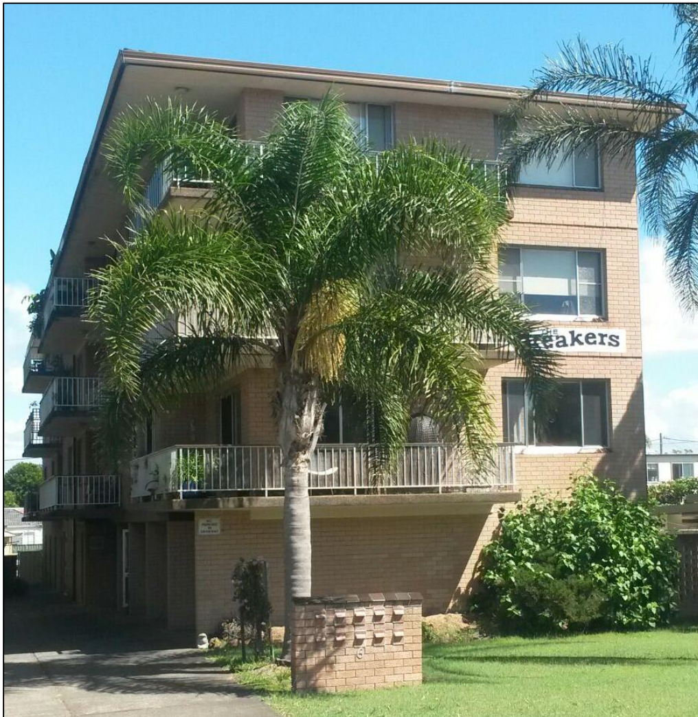
Figure 14 - Existing four storey units in Harrington
