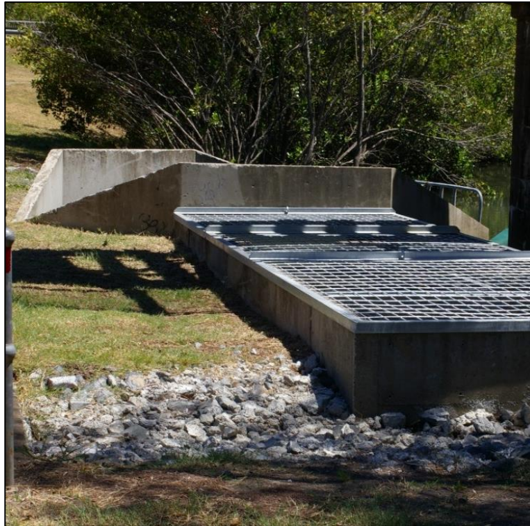
Figure 21 - Renovated Browns Creek Gross Pollutant Trap
