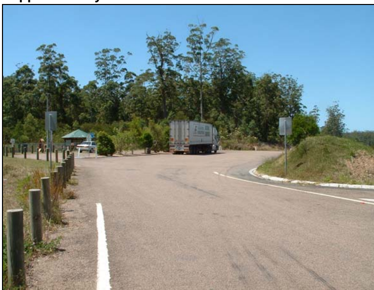
Photograph 2 Rest Area on the Northbound Carriageway of the Pacific Highway approximately 12km to the north of Bulahdelah
