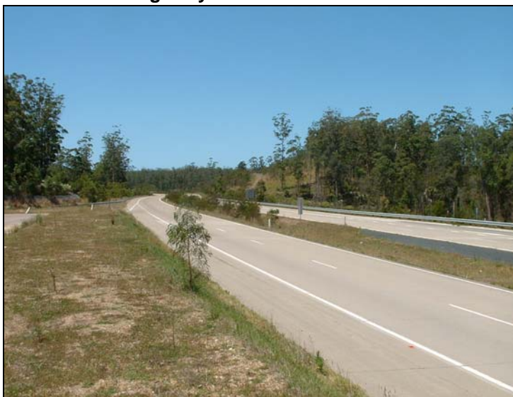
Photograph 1 Looking north along the Bulahdelah to Coolongolook Upgrade section of the Pacific Highway
