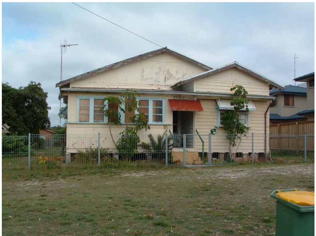
Photo: Site containing old housing stock ready for redevelopment
