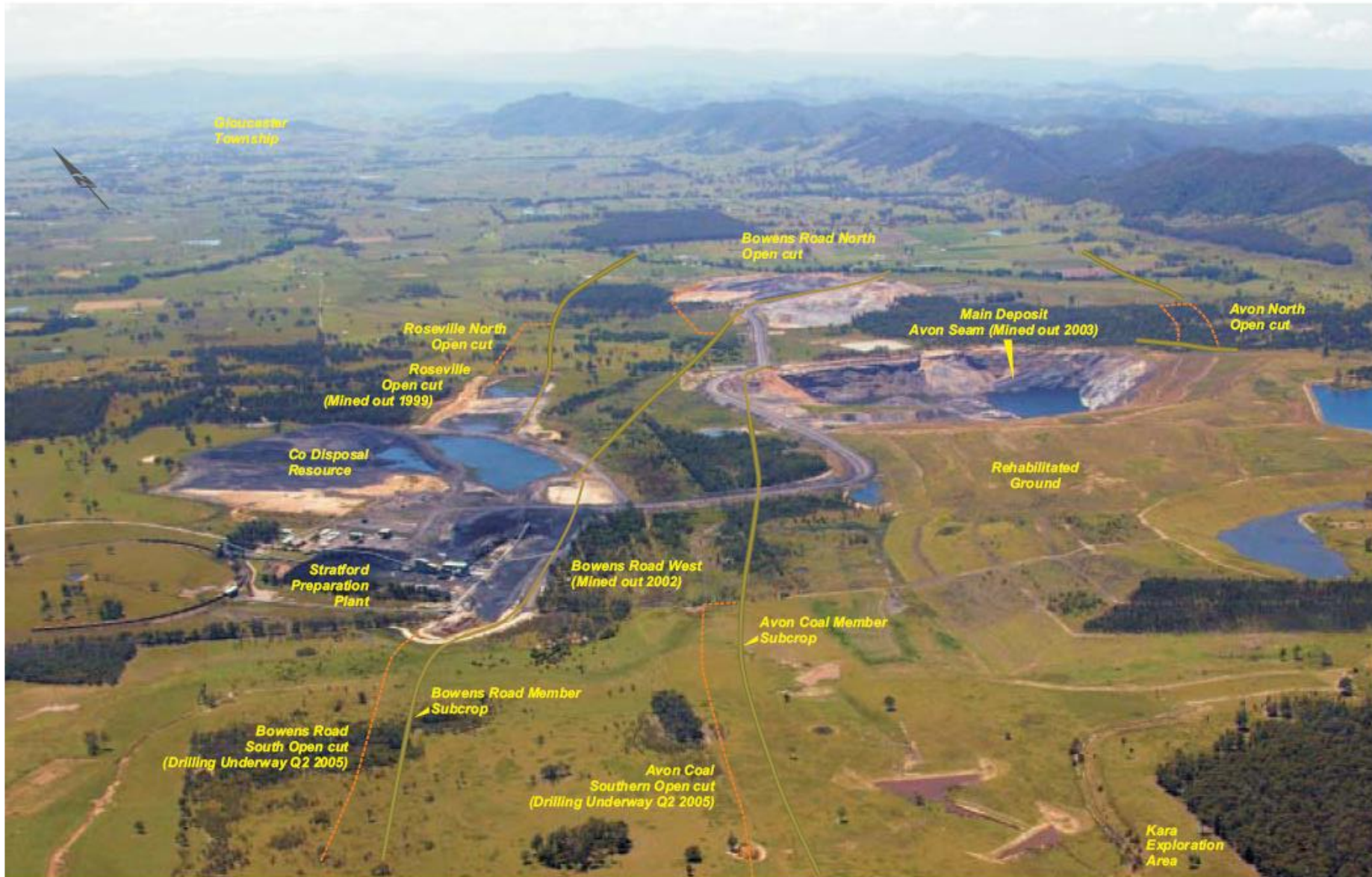
STRATFORD AND BOWENS ROAD NORTH OPERATIONS
