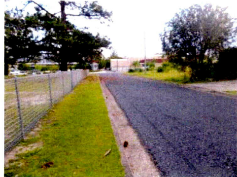
Photo 4: View looking north from the proposed driveway location on Manning Lane.
