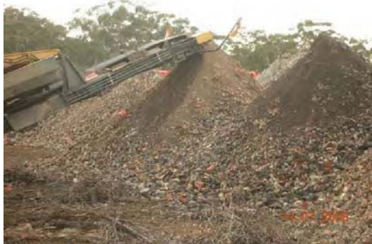
Figure 6.1.2 Concrete crushing (recycling into roadbase) – Tuncurry waste management centre
