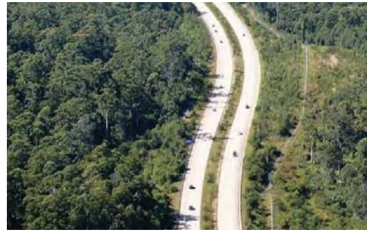
Figure 7.3.1 Roads, such as the Pacific highway, greatly damage and fragment habitat
