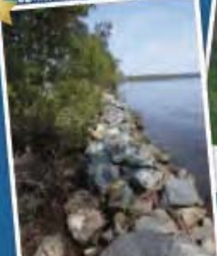
Stabilising 4.2km of the Wallamba River with rock protection, planting 8,000 native plants and conserving 8.6km of streambank
