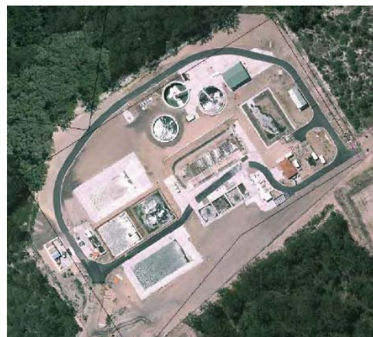
Figure 6.2.1 Sewage treatment at MidCoast Water's Hallidays Point sewage treatment plant.
