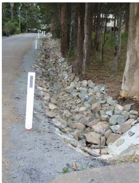
Figure 4.1.18 289 meters of roadside stabilised reducing the amount of sediment reaching the lake
