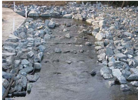
Figure 4.5.1 Remediated Lockett's Crossing fishway. Source: Hunter Central Rivers CMA
