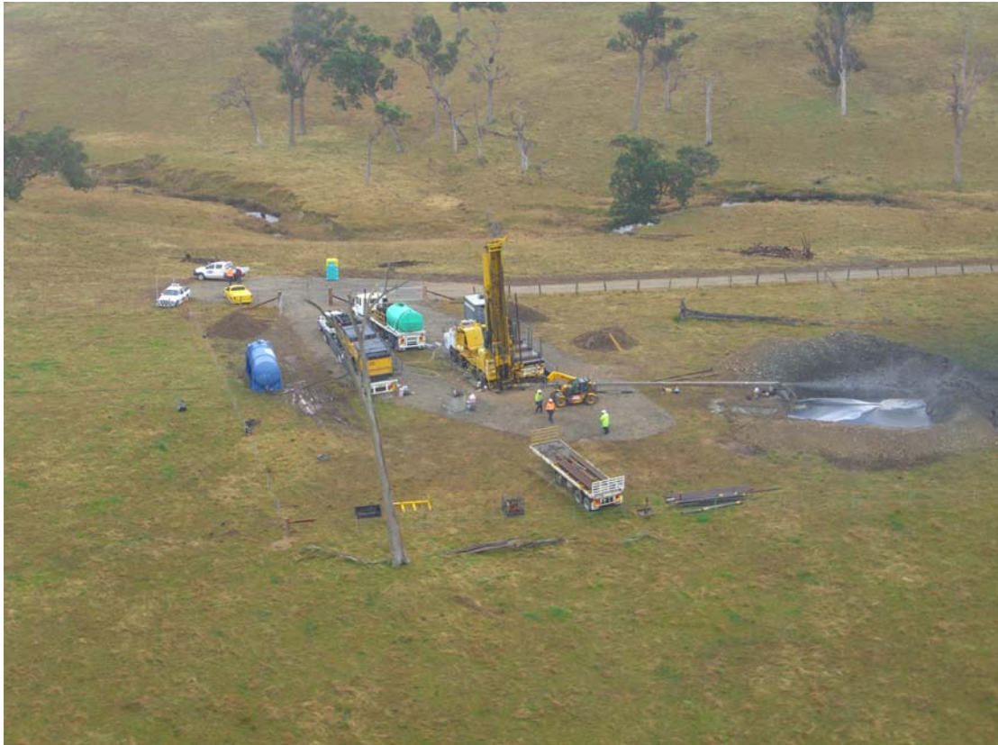
Figure 8. Drill rig in operation adjacent Bucketts Way (Source: Molopo Pty Ltd).
