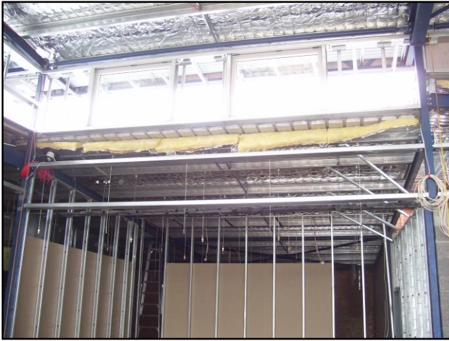
Figure 6. New Council building with installation being installed and high windows for passive solar design, and nearing completion
