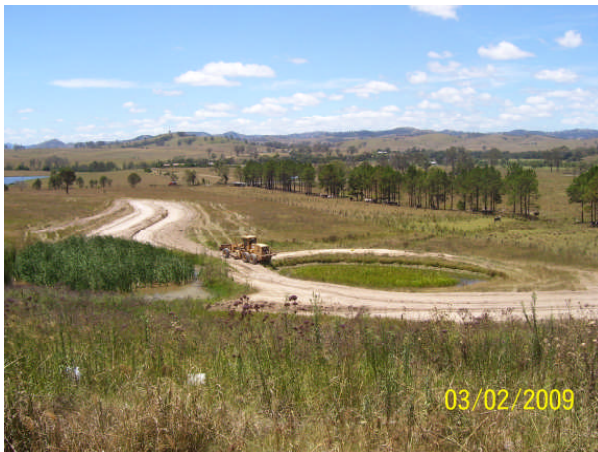
Figure 12 Leachate pond extension
