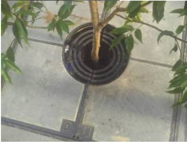
Figure 3.4.5. Dense urban area street tree bioretention.
