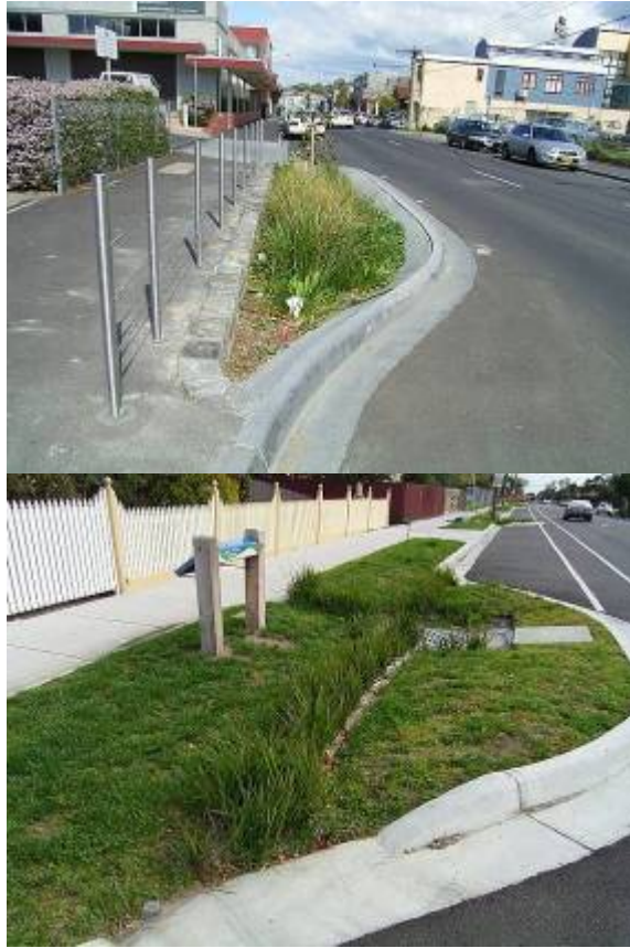
Figure 3.4.6. Street tree bioretention 'pods'.
