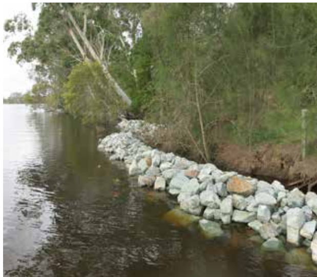
Figure 17: Rock fillets along the Wallamba River
