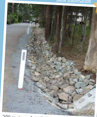
289 meters of roadside stabilised reducing the amount of sediment reaching the lake
