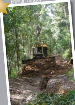
74km roads and trails closed or rehabilitated to reduce erosion and sedimentation in the Myall Lakes National Park
