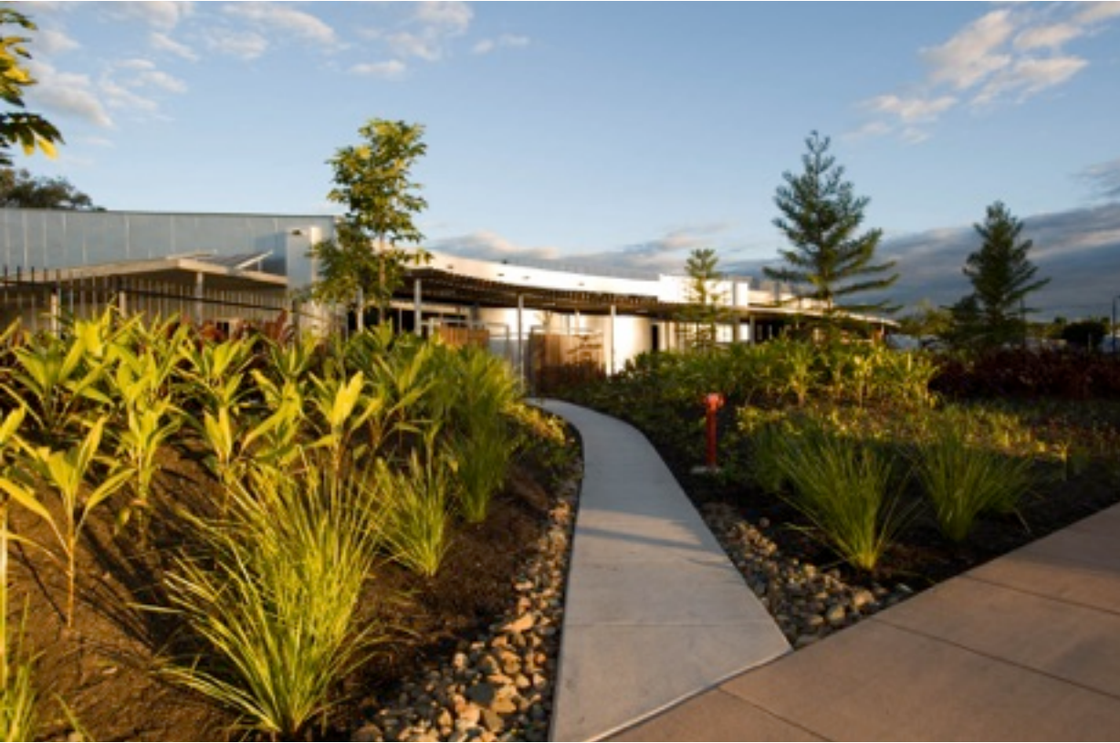
Figure 17: Landscaped forecourt to Cooroy library and digital hub centre
