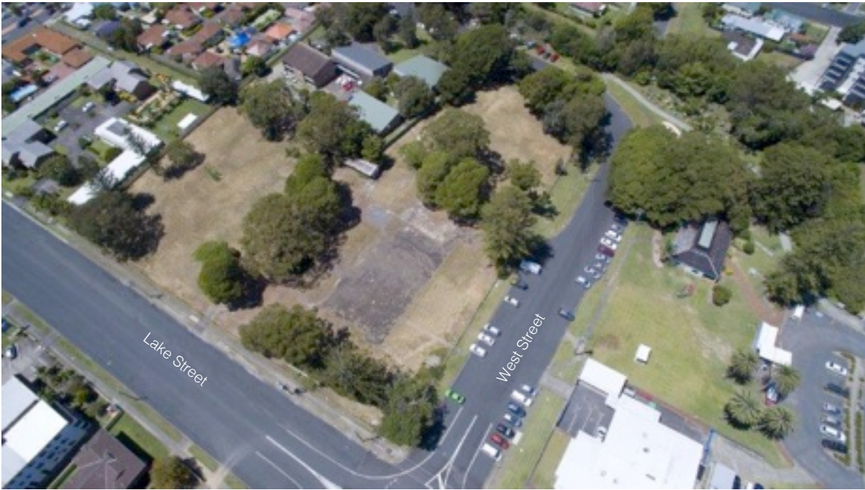
Figure 3: Aerial photo of the site viewed above the corner of Lake and West Streets from the north
