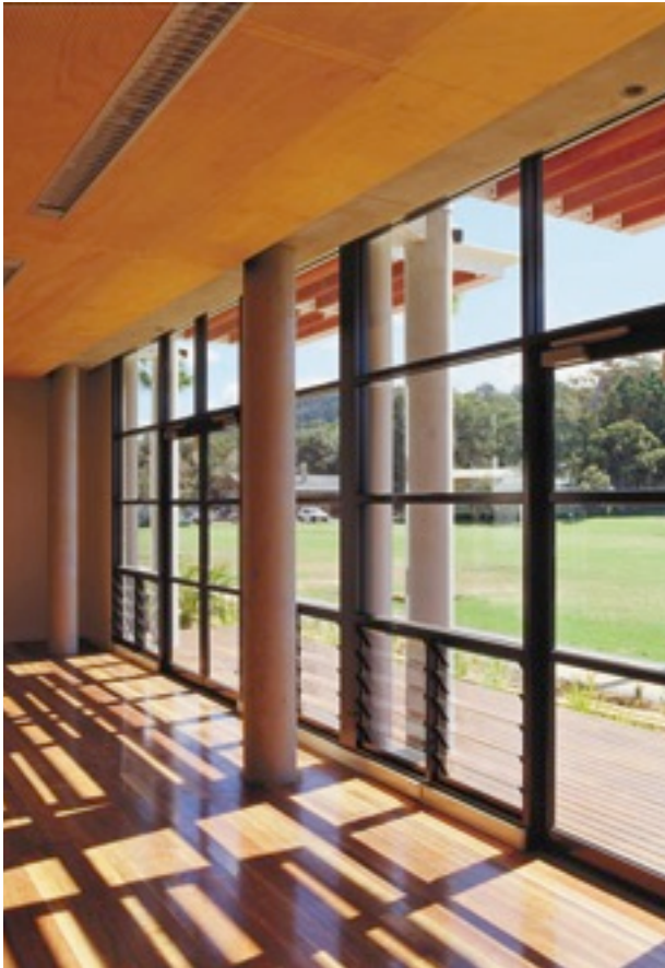
Figure 13: Activity rooms at Avalon community centre connect to adjacent park
